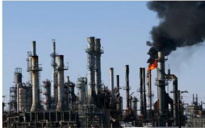
Figure 1 Industrial Steel Chimneys (Ref: www.vedomosti.ru )
